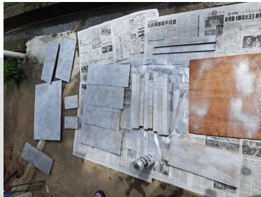
Figure 3: The plywood Spraying Process
